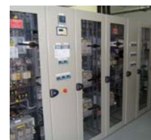
Pre-cabled distribution board
